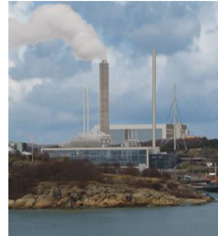
GoBiGas Phase 2 80-100 MW bio-methane Commercial Plant
