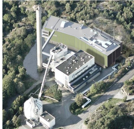
GoBiGas Phase 1 20 MW bio-methane Demonstration plant
